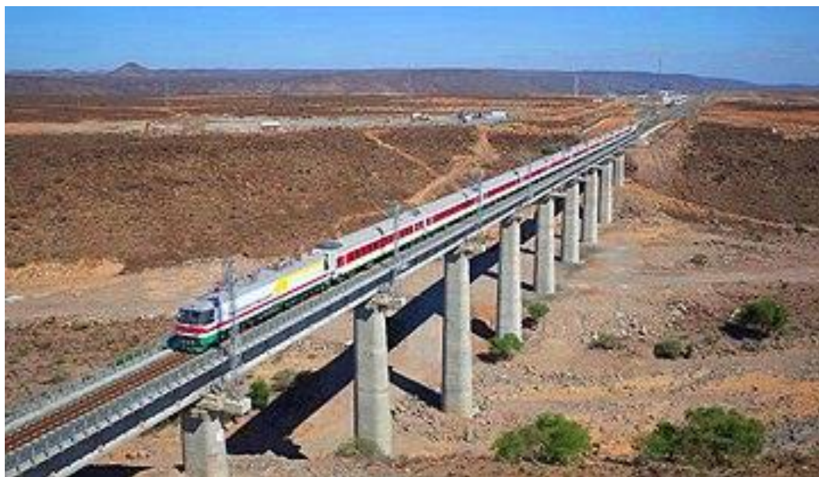
Figure 0-1: Holhol Bridge on the Addis Ababa-Djibouti Railway
